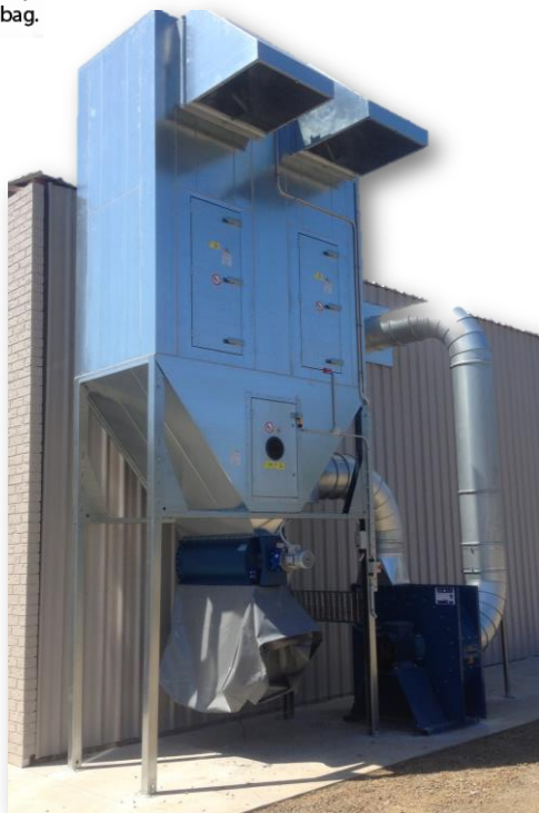
1HJ with 2 x Regeneration cleaning fans
